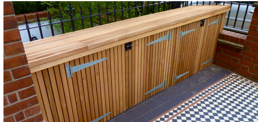
Figure 2 Example of covered cycle storage
